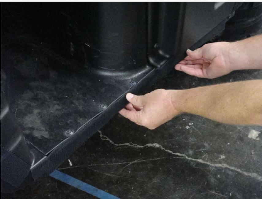
Figure 5.1 – attach 27” Velcro Strips horizontally along the door Rocker Panel – align the top side and fold the bottom 1” underneath the Rocker Panel
